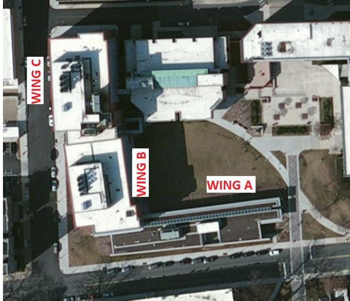
Figure 3: Wings A, B, and C of S.T.E.P.S. Building
